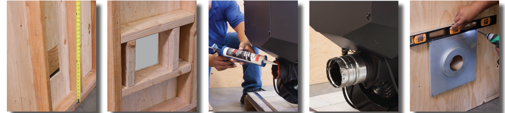
1. Locate appliance and penetration through wall.
