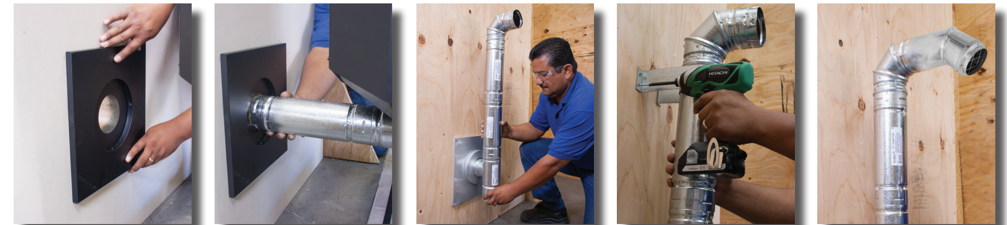
6. Level and attach inside portion of the wall thimble to the wall.
