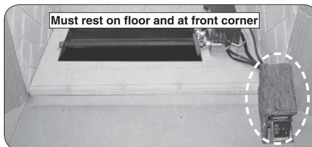
Fig. 10-2 Place heat shield
